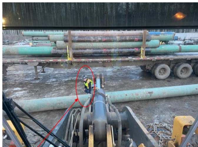
Loader operator's field of view and position of the injured worker
