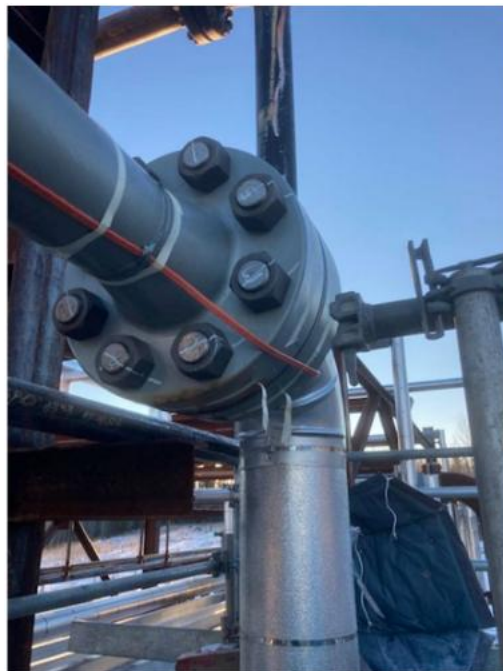
Figure 1: Flanged connection
