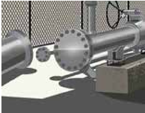
Figure 3-7: Blank or Blind
