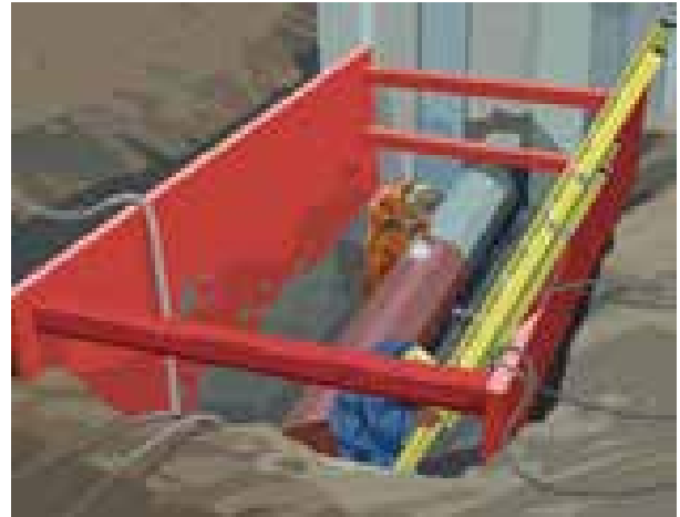
Figure 4-13 Trench Shield
