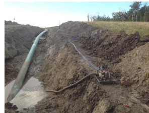
Excavation that was being dewatered. Water was being pumped up hill.
