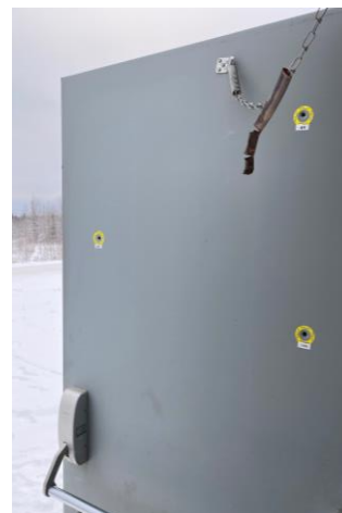
Bullet holes in the wall and door of the compressor building
