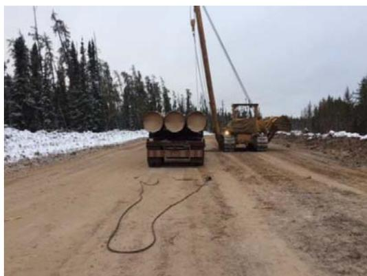
**Broken Hoist Line on the Ground**
