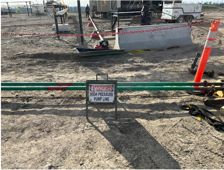
Figure 52. Service Rig Exclusion Zone Example
