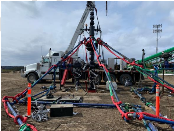
Figure 4. Restraints Used During Fracture Operations
