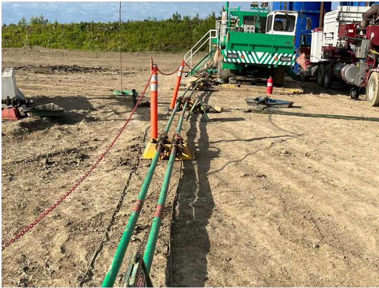
Figure 53. Service Rig Exclusion Zone Example
