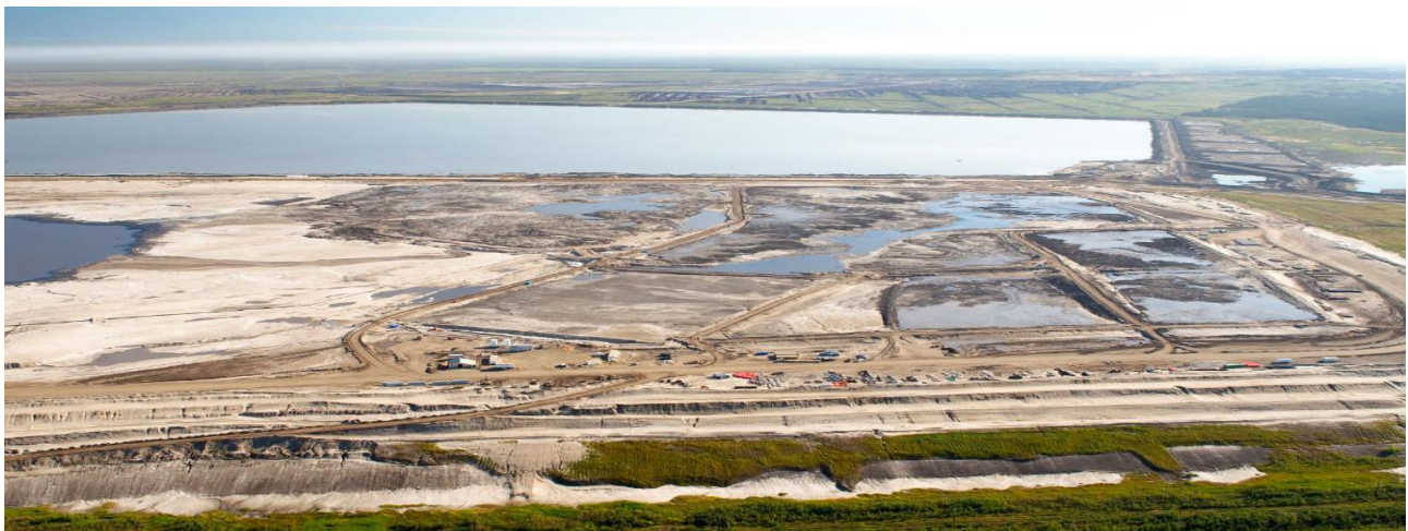
Aerial photo of an oil sands tailings storage facility. Source: osqar.suncor.com
