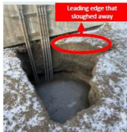
Opened hole after hydrovac operation 1m x 1.5m x 1.5m
