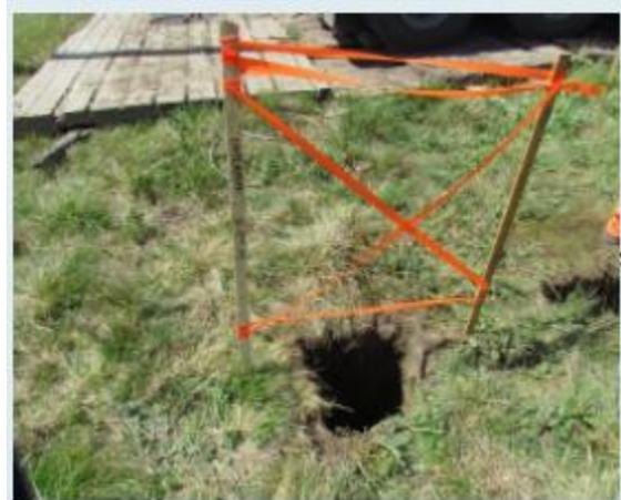
Typical hydrovac daylighting (~1m)
