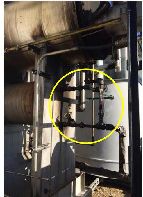
**Scorched Piping/Insulation Under Reboiler**
