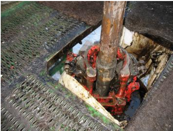
Photo 1: Position of Slips Under Service Rig Floor
