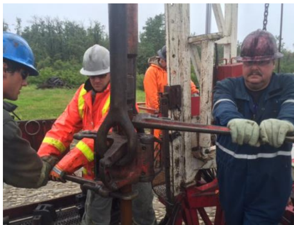
Re-enactment of workers torquing tubing with pipe wrenches
